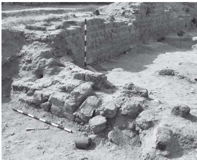
Fig. 5. Entrance wall to the courtyard.
